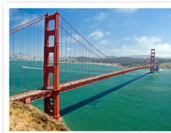
Golden Gate Bridge
